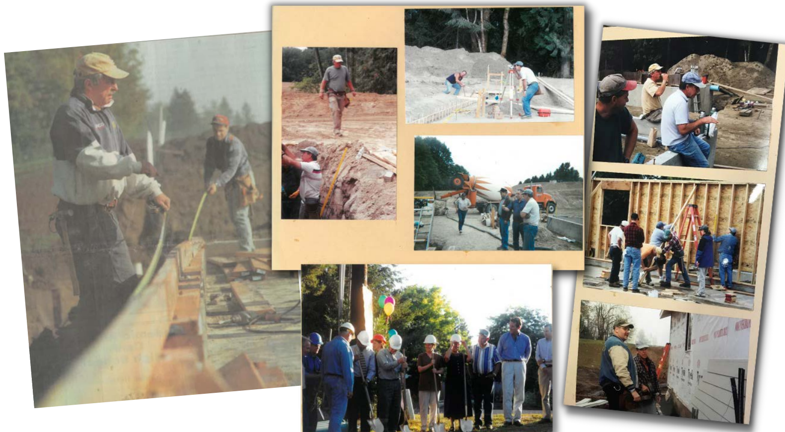
Community volunteers building our wastewater system after the 1997 bond passage.
