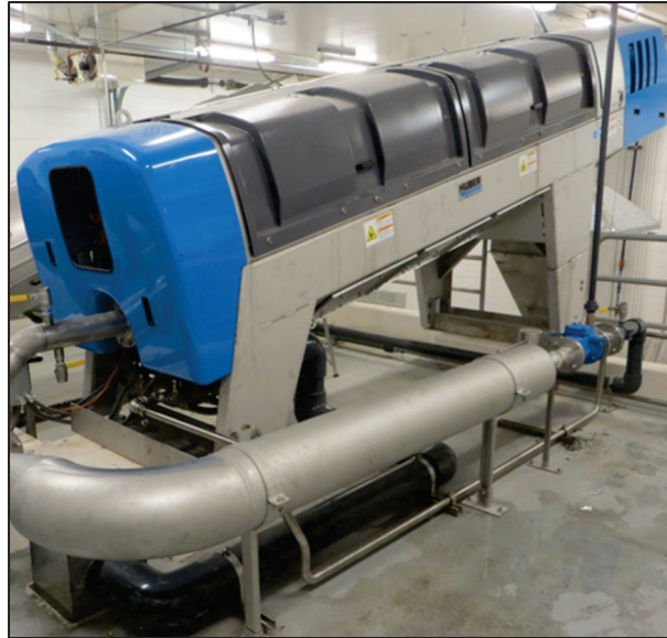
FIGURE 4-6: SCREW PRESS
